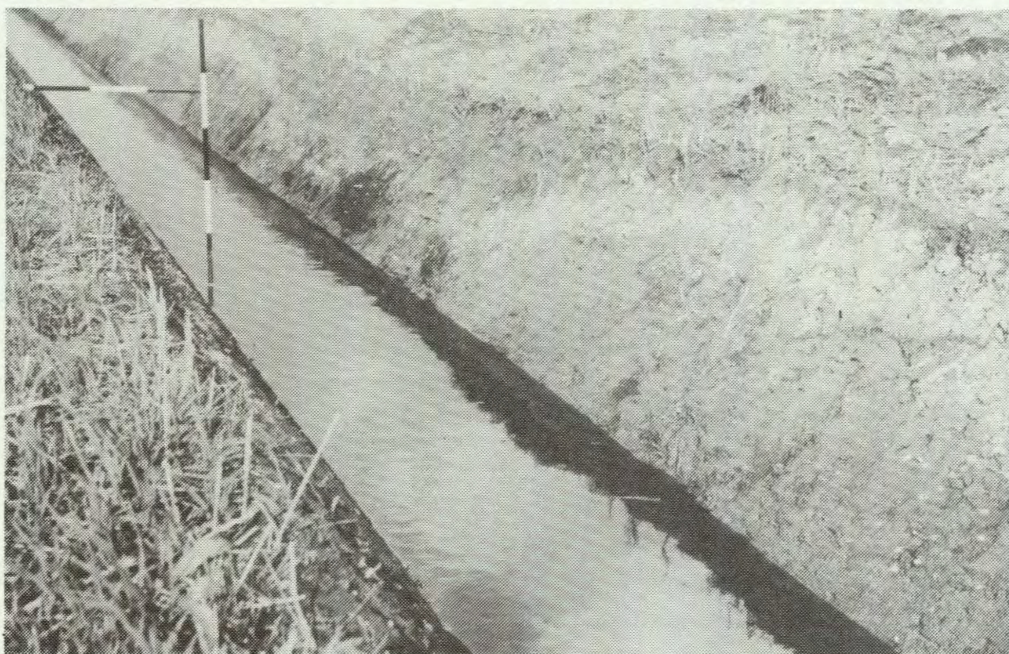
The undulations of the clay subsoil can be clearly seen in this exposed dyke bank. Photograph courtesy of the Arthur Rickwood EHF.
