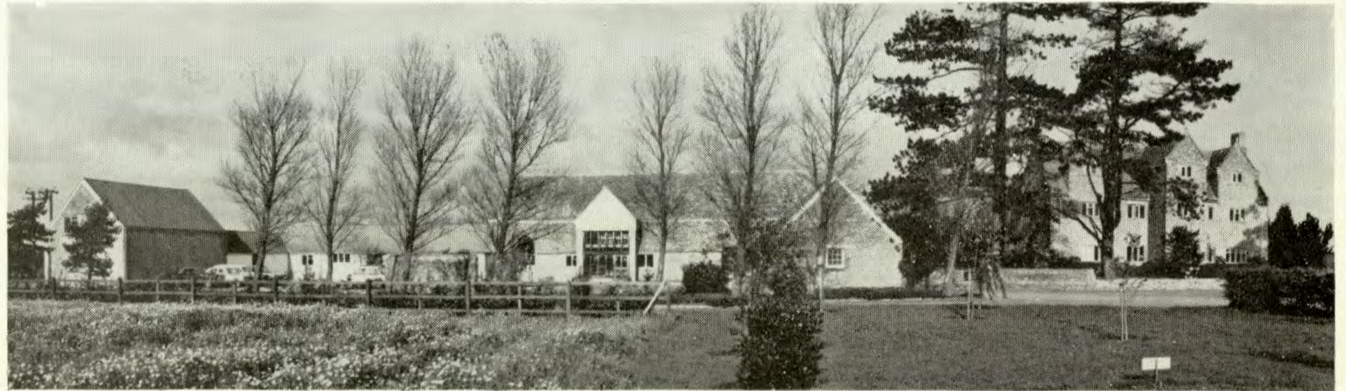
General view of the old buildings from the South.
