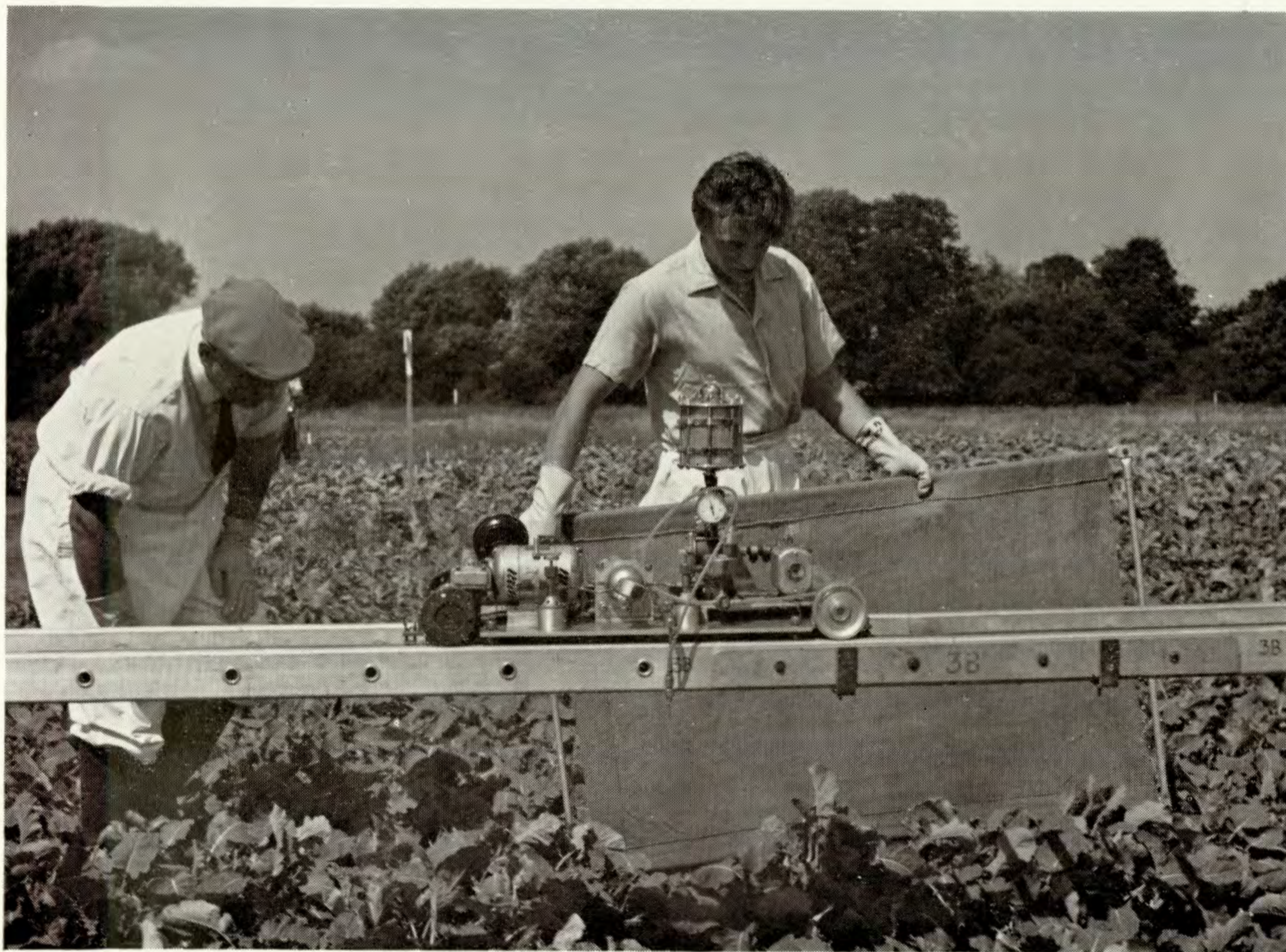
Field testing of herbicides with the W.R.O. Logarithmic Sprayer
