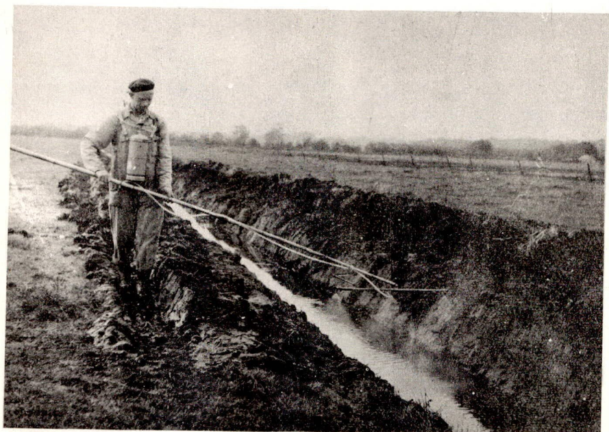
FIG. 3. PROPANE KNAPSACK SPRAYER
